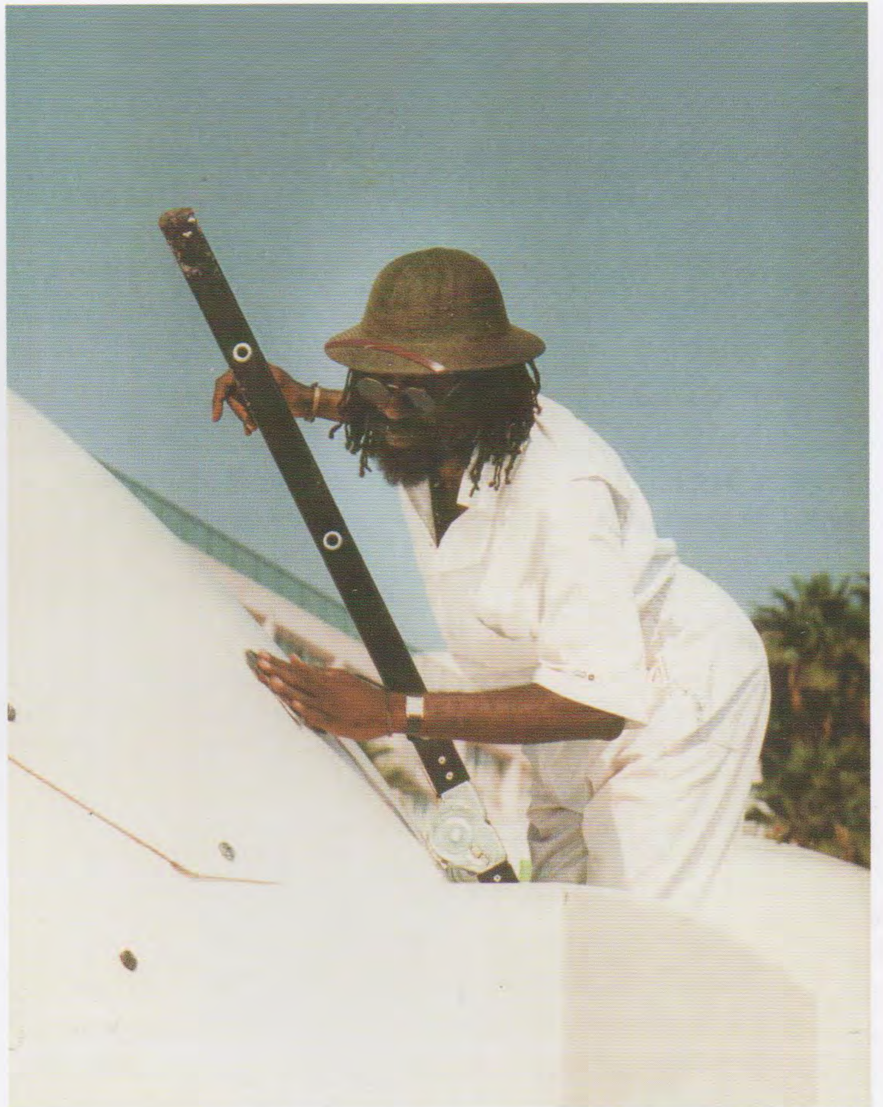
Above: Ted constructing Dome Village circa 1993.
